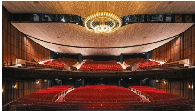
Above: In the renovated hall at Théâtre de Beaulieu in Lausanne, Switzerland, the new timber ceiling is higher than previously and curved to provide early sound reflections to all audience areas
